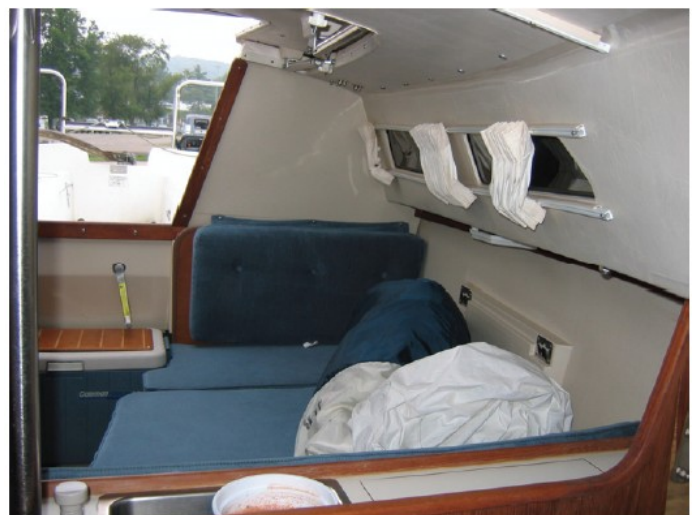
On the bottom right of this photo, you can barely see that there is some veneer missing from the area near the chain plate bolts.
